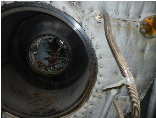
Pic showing in field receiver ring installation
