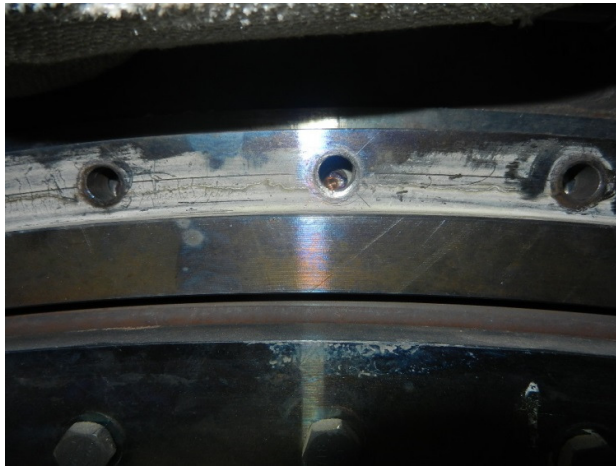
Pic showing in field receiver ring installation
